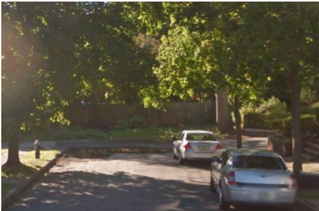
The dead end at Warman Street, circa 2013, with the sort of puddle a new drainage project is meant to alleviate. Image courtesy of Google.
